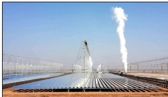
Fig 9: Plant in Rajasthan[17]
