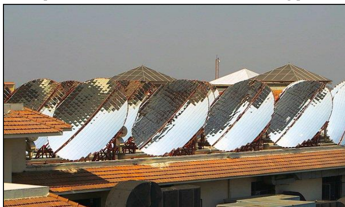
Fig.13 Dish collector plant (PC shirdi sansthan, Maharashtra)
